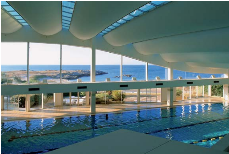
Work is currently underway on the renovation of Thalassa's 5,000sq m flagship property in Quiberon in north-west France
